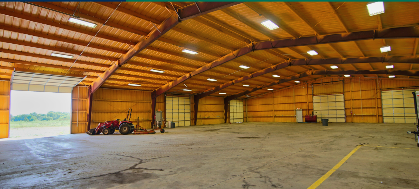
Interior of Warehouse Building
